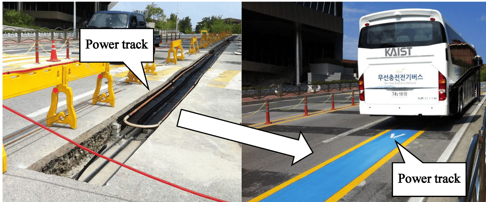
(a) DWC-EV power track under construction
